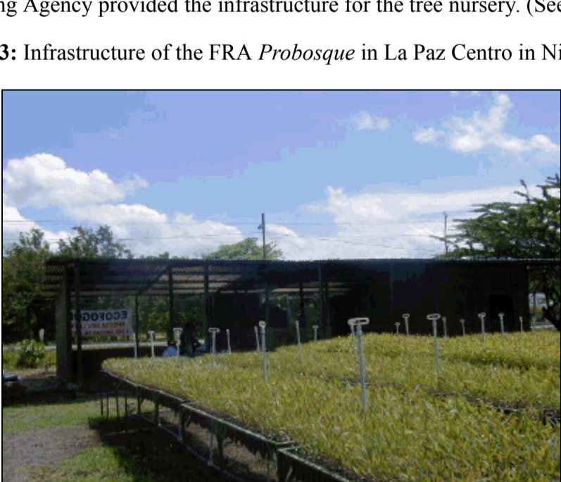
Picture 3: Infrastructure of the FRA Probosque in La Paz Centro in Nicaragua.
